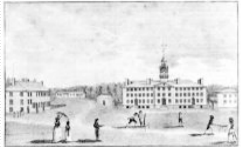
A first View of DARTMOUTH COLLEGE, with the FRANKLIN'S HALL.
