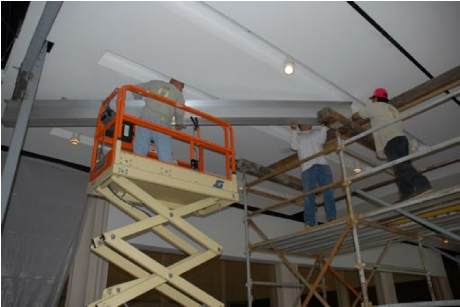
Installing the I-Beams
