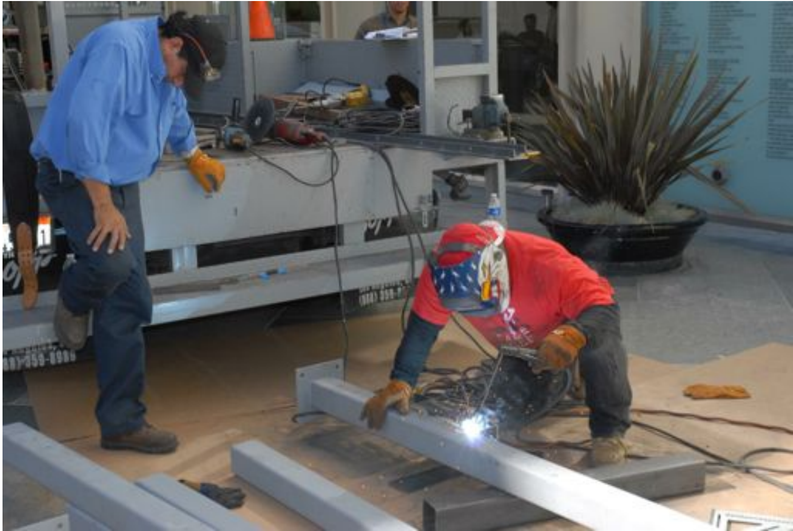
Fabricating the metal frame on site
