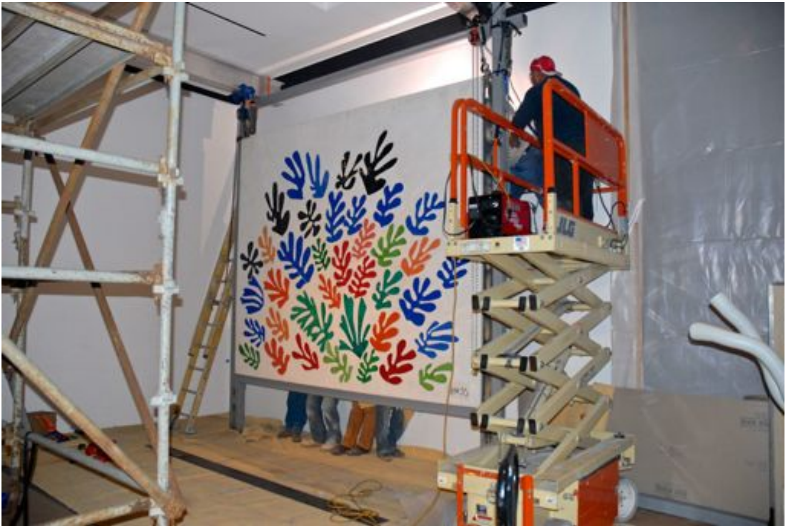
Welding the Matisse to the steel frame
