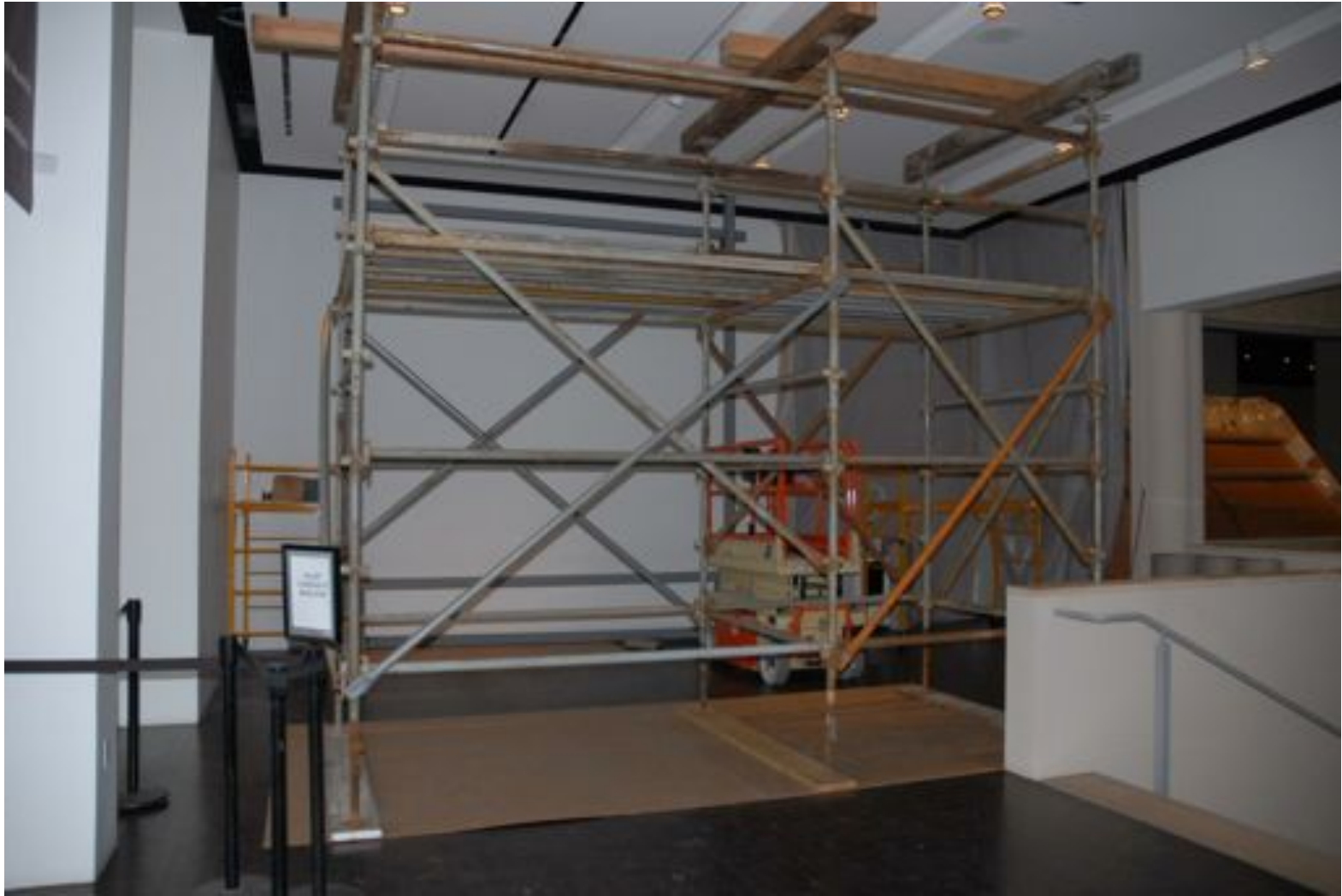
Scaffolding for the I-Beam support
