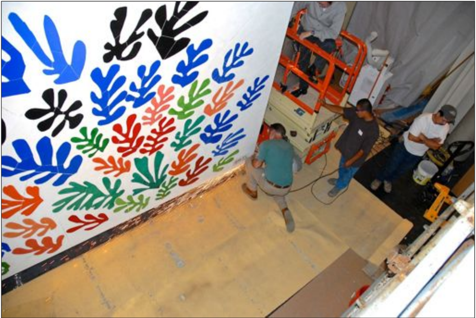
Adjusting the steel support
