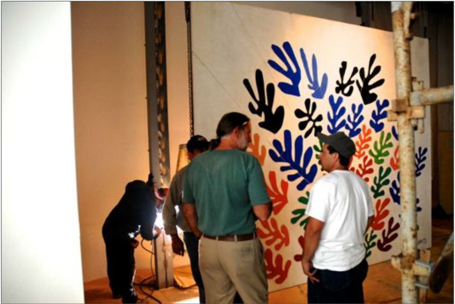
A welder adjusting the steel support
