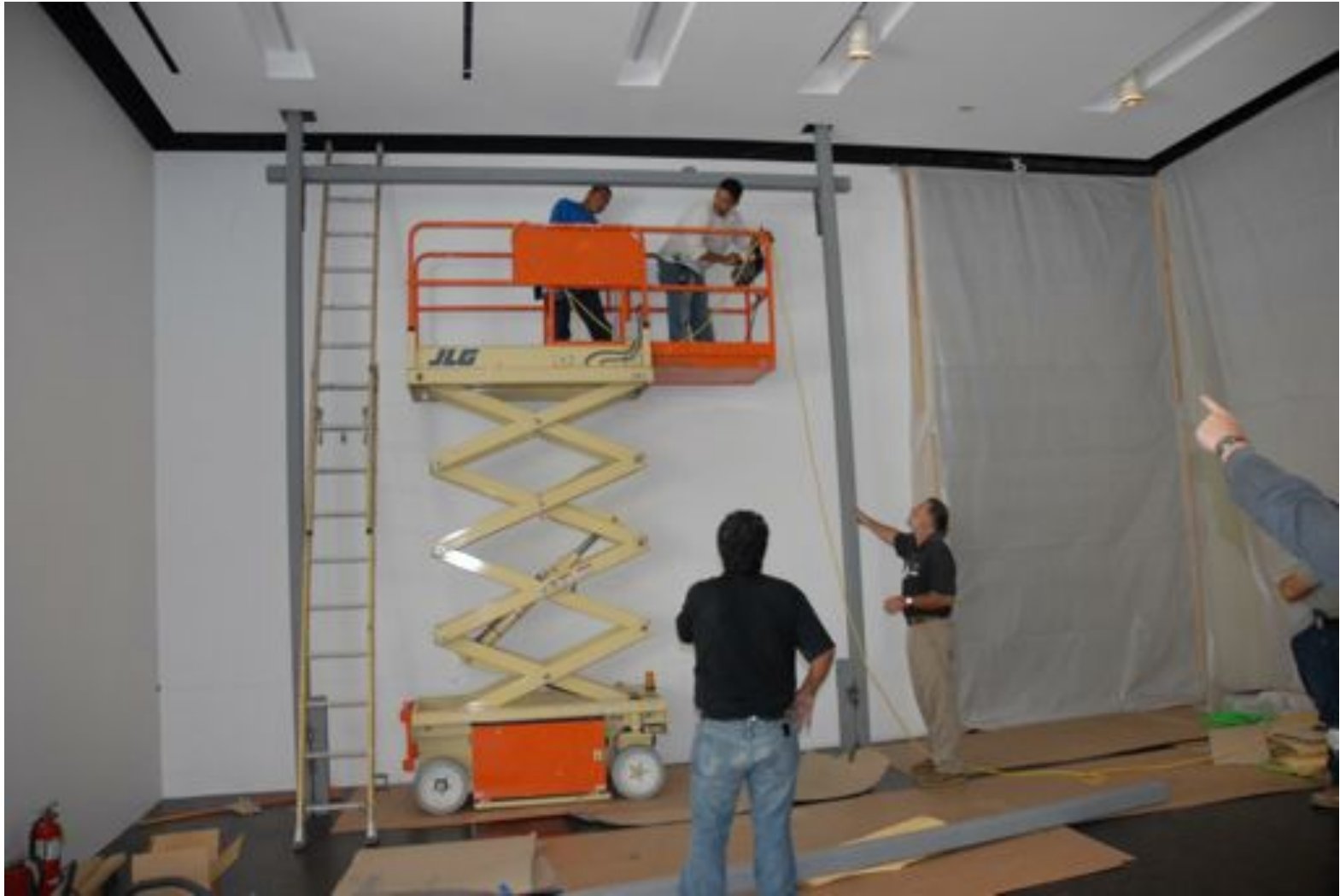
Installing the I-Beams support
