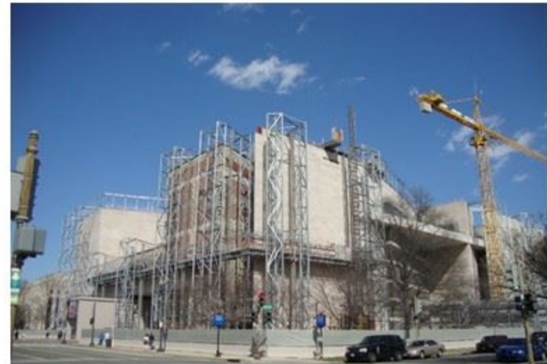
East Building renovation 2013-present
